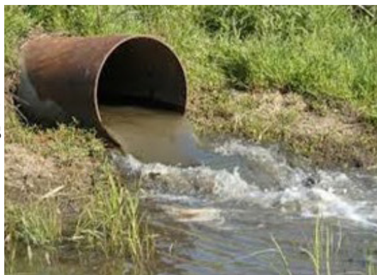
Figure 7.1 Air pollution caused by industrial waste
